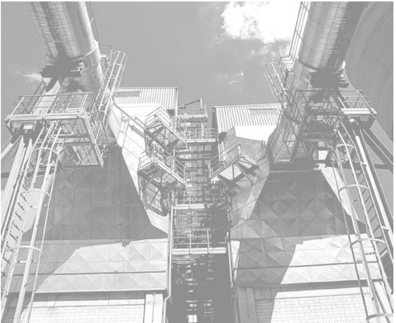
Flue gas treatment devices of a cement kiln
