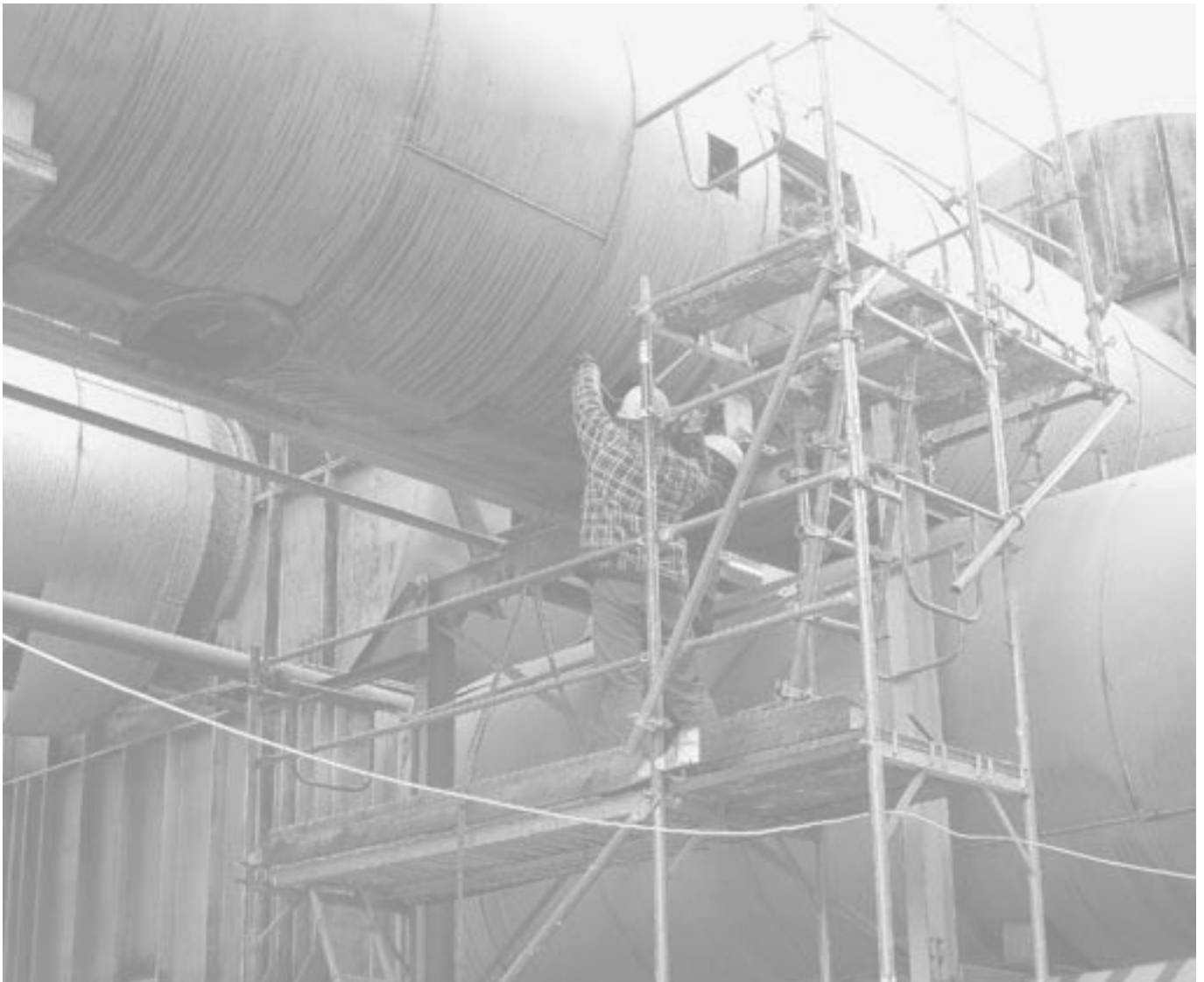
Safety at maintenance according to regulations
