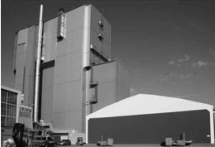
Fig. V-44: AVR experimental reactor with material lock (left) and construction site tent to fill the reactor chamber (right)
