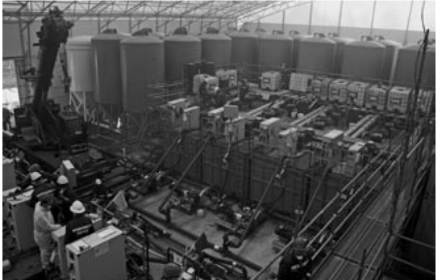
Fig. V-45: View of four of the eight mixing tanks, some of the silos containing constituents and the mobile crane inside the construction site tent
