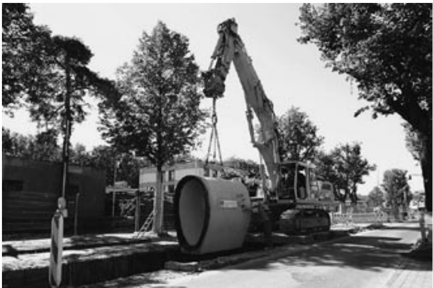
Fig. V-61: Laying of concrete pipes for the effluent domain
