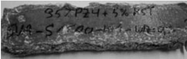
Fig. III-29: Flat mortar prism made from Portland cement (CEM I 32.5 R containing 5 mass % limestone meal as a minor additional constituent) after 24-month storage in sodium sulphate solution (1500 mg SO 4 /l) at 8 °C
