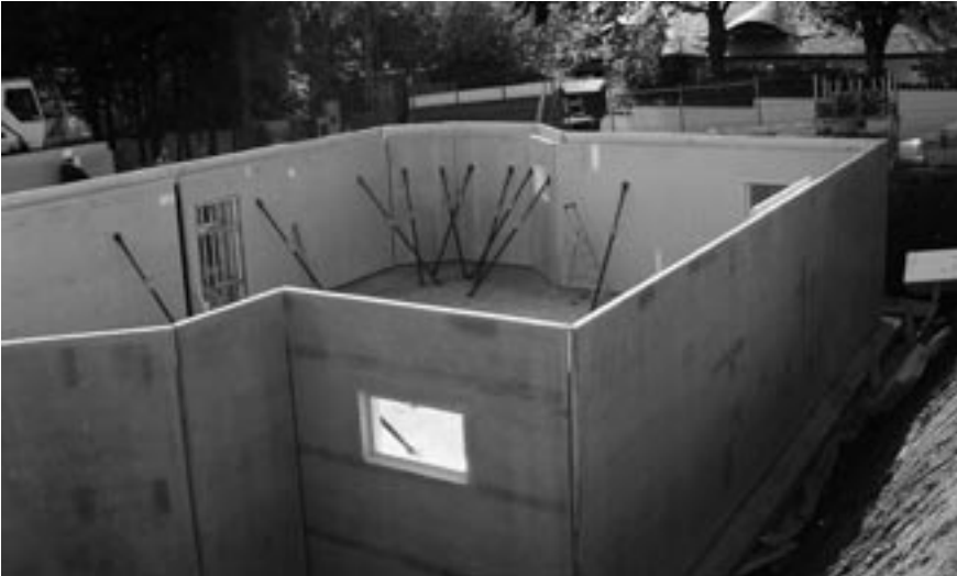
Fig. V-59: Erection of a waterproof concrete basement (water-impermeable concrete)
