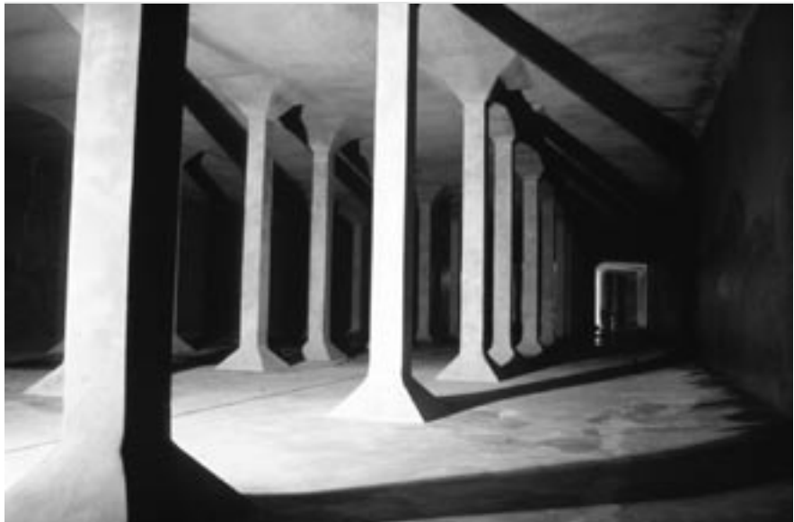
Fig. V-60: Drinking water tank after repair
