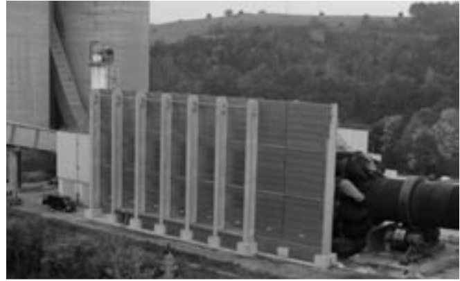
Fig. II-27: Situation after erection of the sound screen
