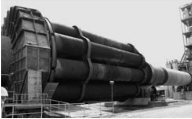
Fig. II-26: Situation before erection of the sound screen
