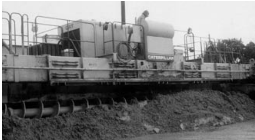
Fig. V-19: Spreading by slip form paver: mixing energy is applied to the fresh concrete by the distribution screw
