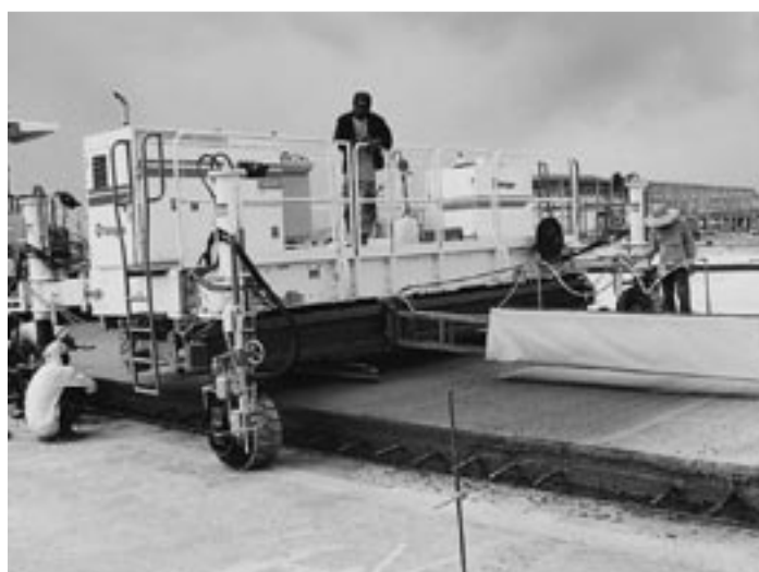
Fig. V-34: Spraying of the curing agent by an automotive device
